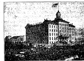
Hough House erected in 1896 at a cost of $125,000.00. Was located on the southeast corner of the Stock Yard Grounds. At the left of the picture is shown the scales on which cattle were weighed and brought in for butcher or sale. Hough House was famous rendezvous for stock traders.
