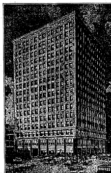
Kimball Hall Building. Executive offices and sales rooms of the Kimball Piano Company.
